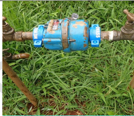
Figure 8.12: Meter Sealed Using Plastic Seals
