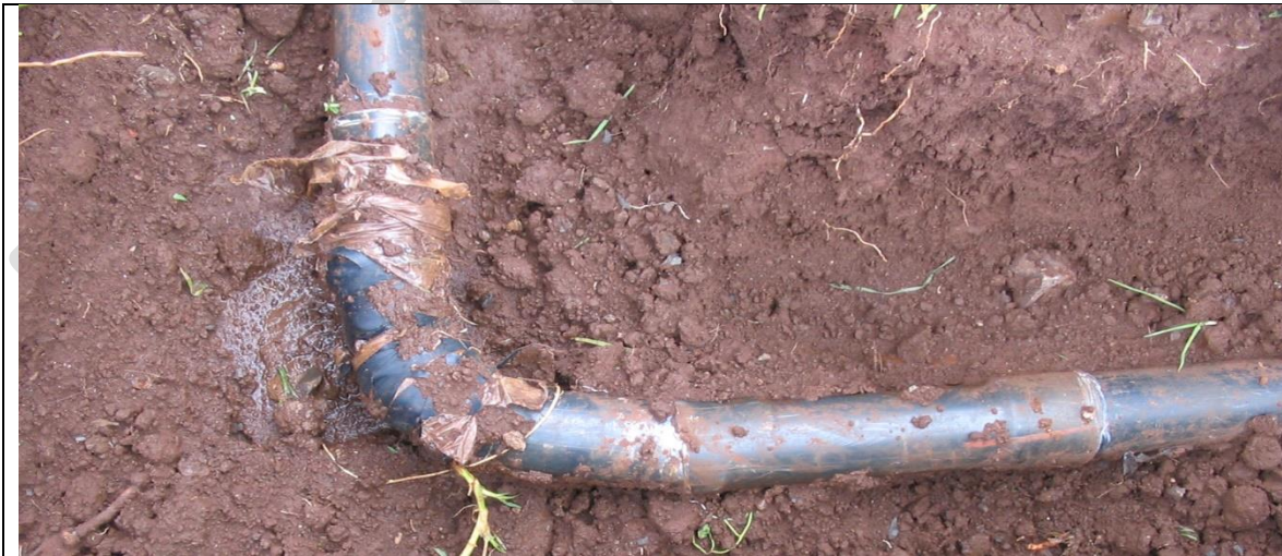
Figure 2.15: Poor Repairs with Fire-made Couplings
