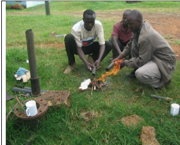
Figure 2.13: Softening Pipe by Heating
