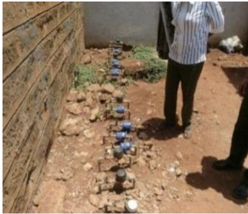
Photo 3.1: Installation of Customer Meters without meter box
