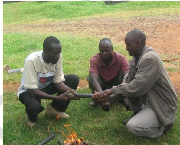
Figure 2.14: Making Fire-made Coupling from Softened Pipes
