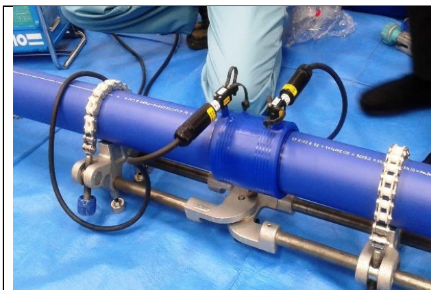
Figure 2.25: Electrofusion Welding in progress
