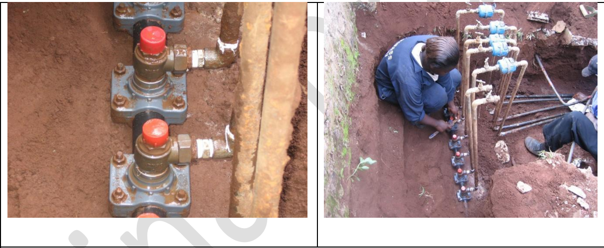
Figure 3.1: Tapping with standardized saddle clamp and ferrule (tap)
