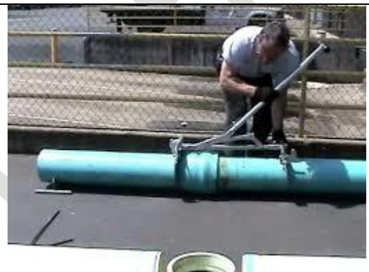
Figure 2.12: Pipe puller
